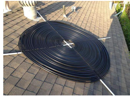
Figure 2.2: Polyethylene tube arrangement
