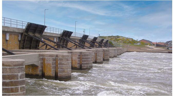
Figure 1: Storm surge barrier at Hvide Sande (from [2])
